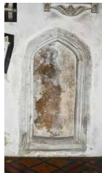
A former doorway, probably bricked up in 1712.
